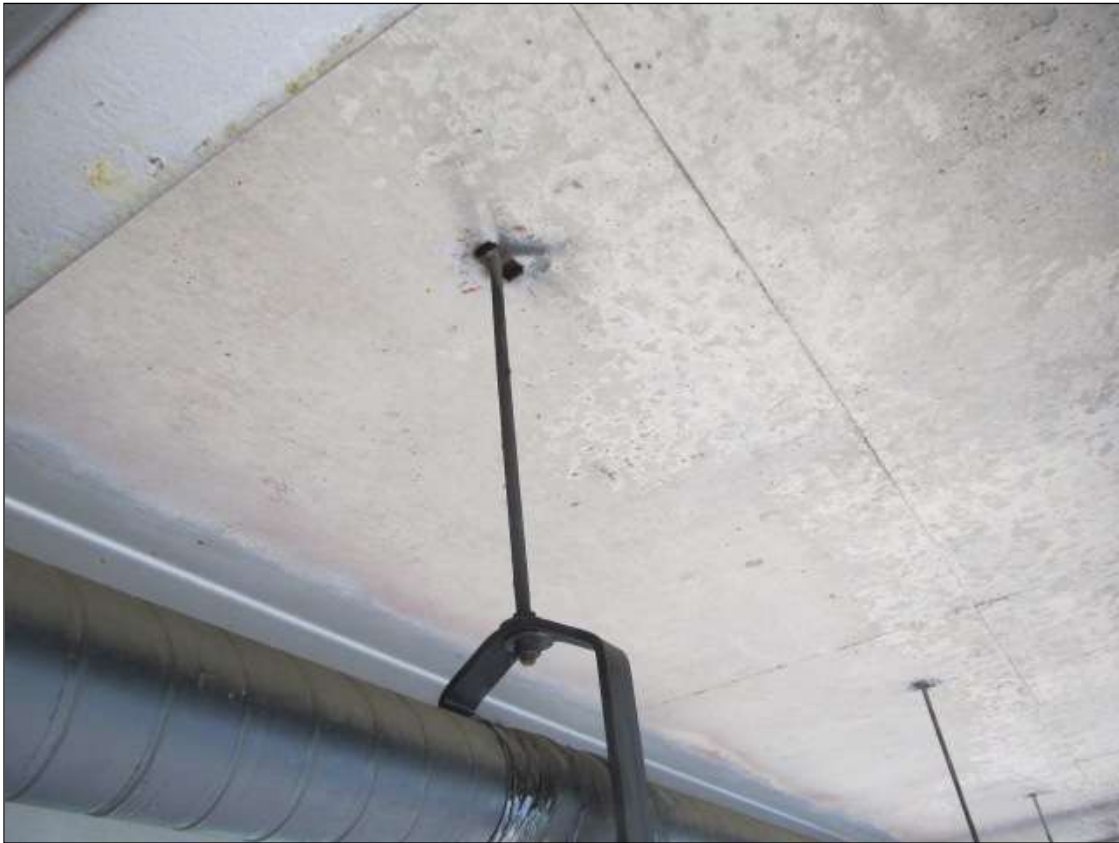
UTILITY HANGER FOR GAS LINE
