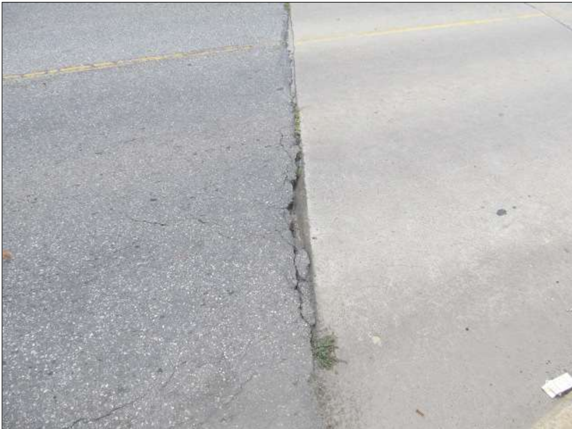
ASPHALT CHIPPING ALONG THE APPROACH SLAB AND RDWY. FOR TE WEST AND EAST APPROACHES
