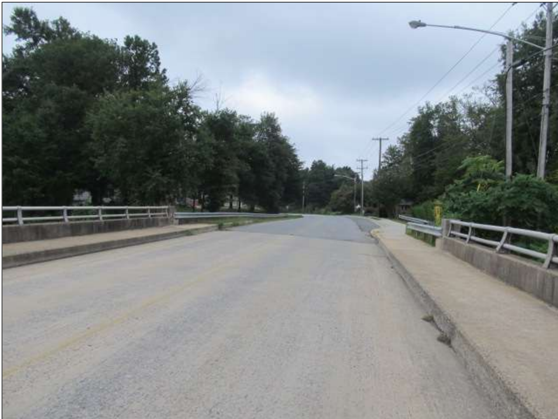
GUARDRAIL LOOKING EAST
