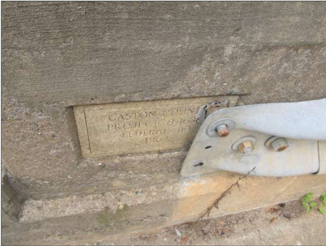
DIAG. CRACKING ALONG THE END SPANS.
