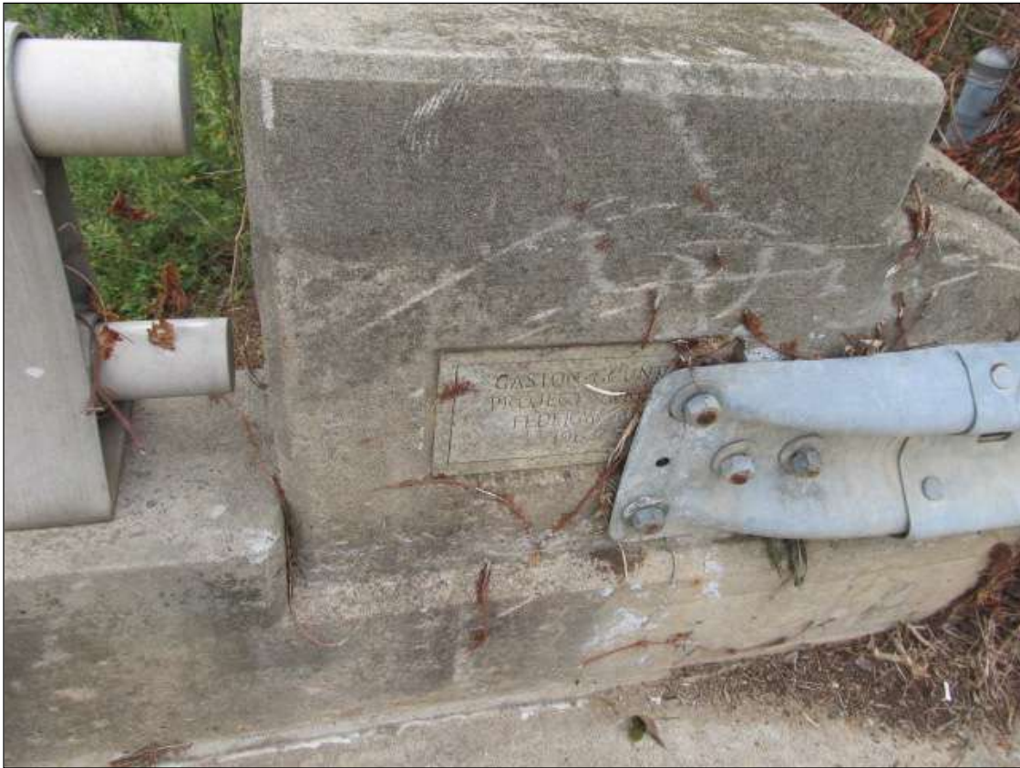
BRIDGE INFOR. PLATE FOR THE NORTHEAST AND SOUTHWEST CORNERS (NORTHEAST SHOWN)
