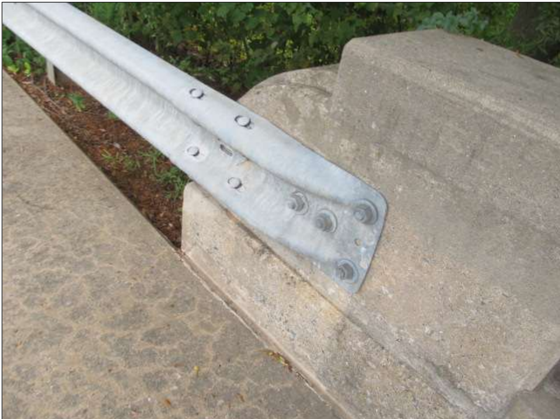
GUARDRAIL ATTACHED TO THE BRIDGE RAILS FOR ALL FOUR CORNERS (NORTHWEST SHOWN)
