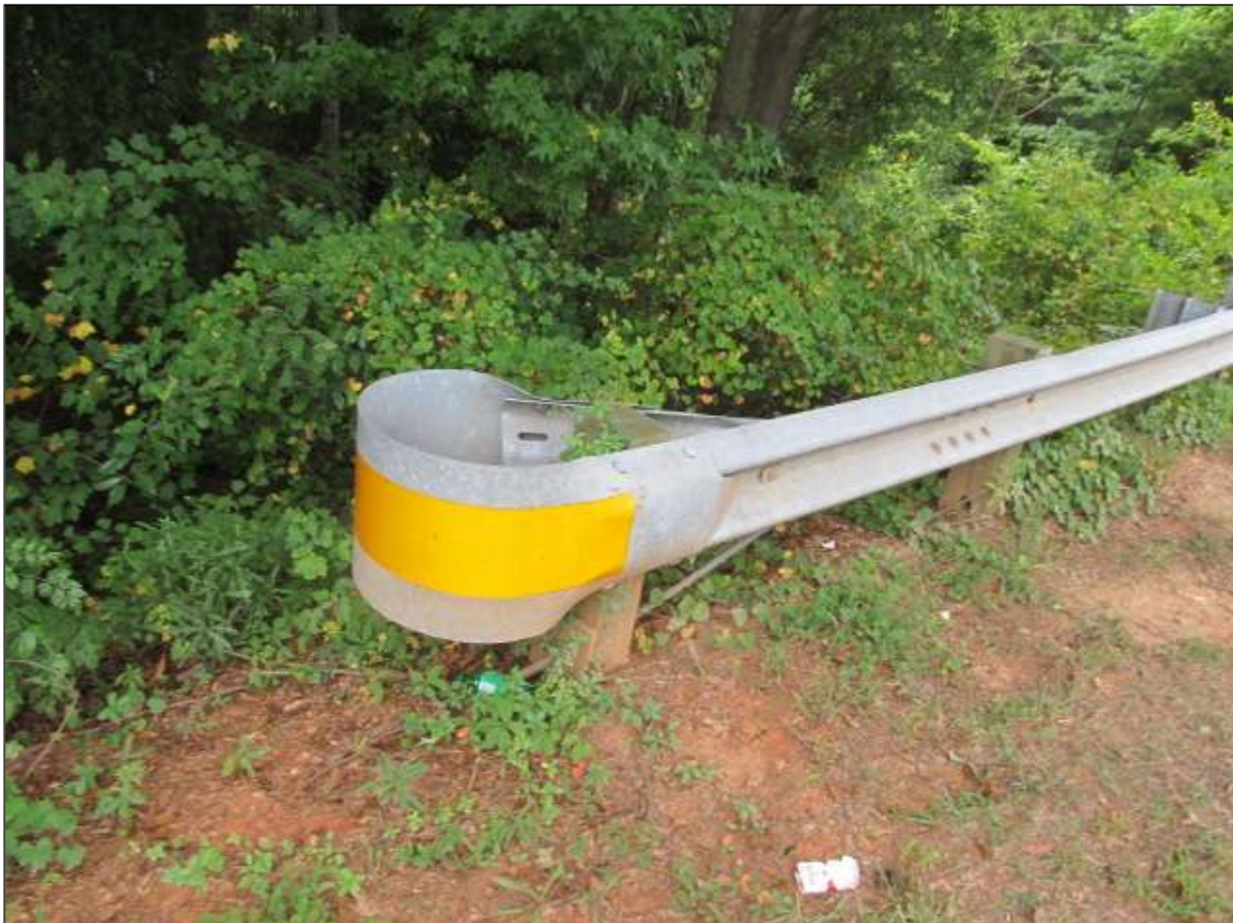
GUARDRAIL END FOR ALL FOUR CORNERS NORTHWEST SHOWN
