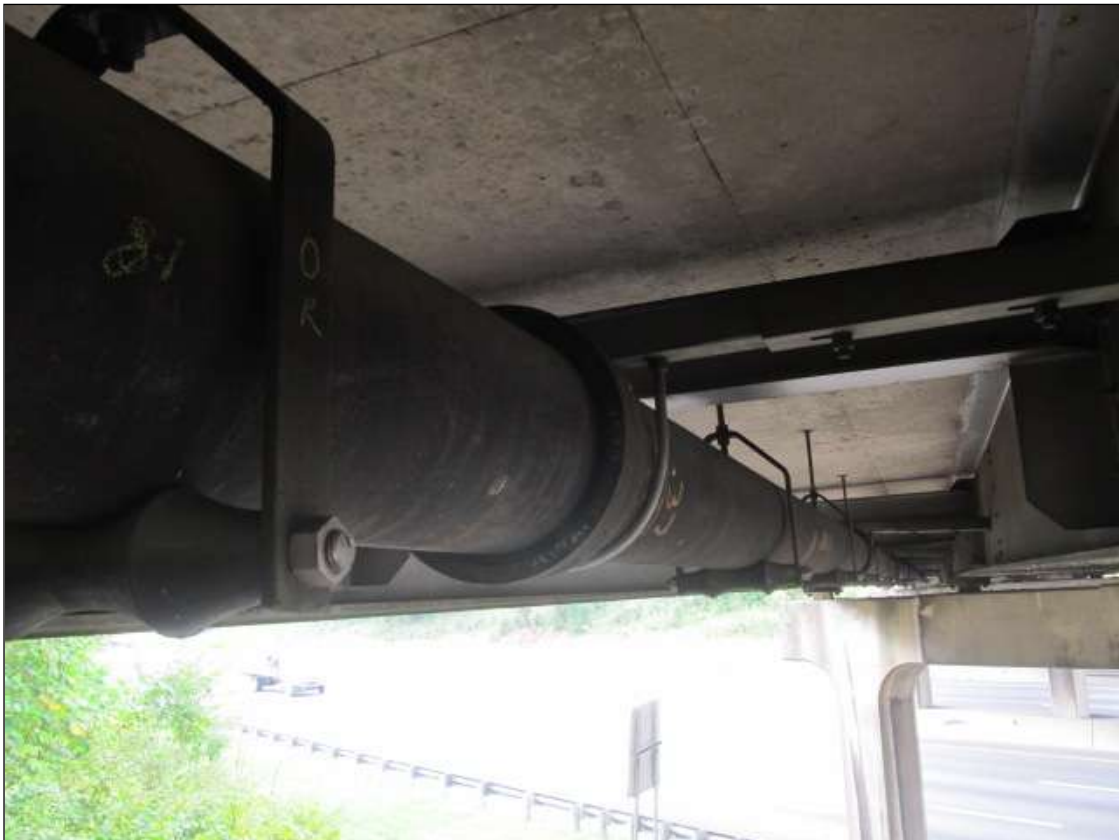
UTILITY UNDER BAY 1
