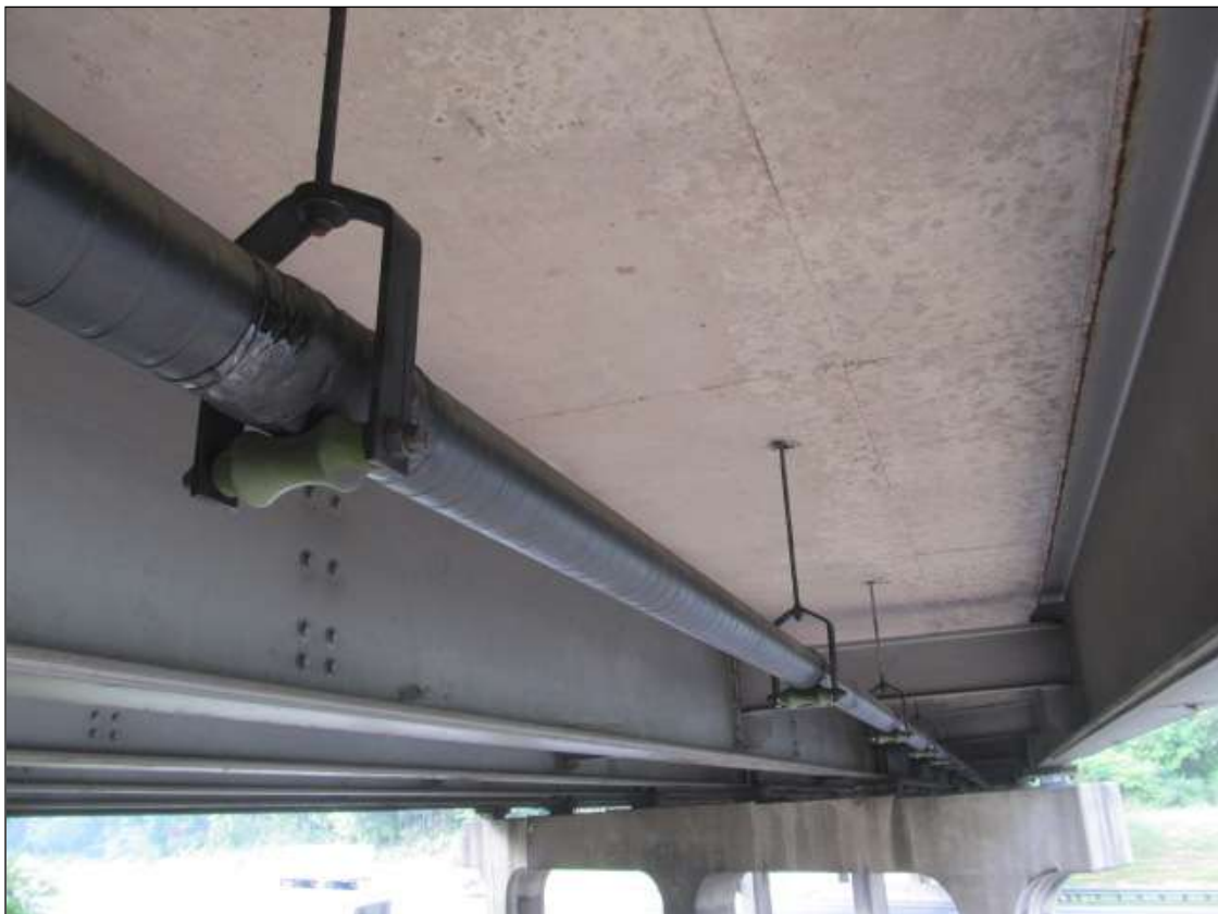
GAS LINE UNDER BAY 5
