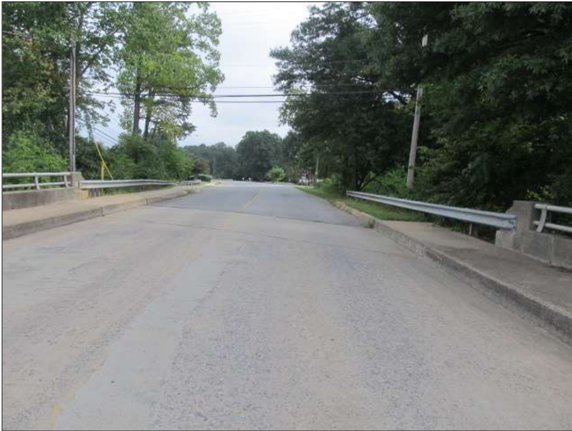
GUARDRAIL LOOKING WEST
