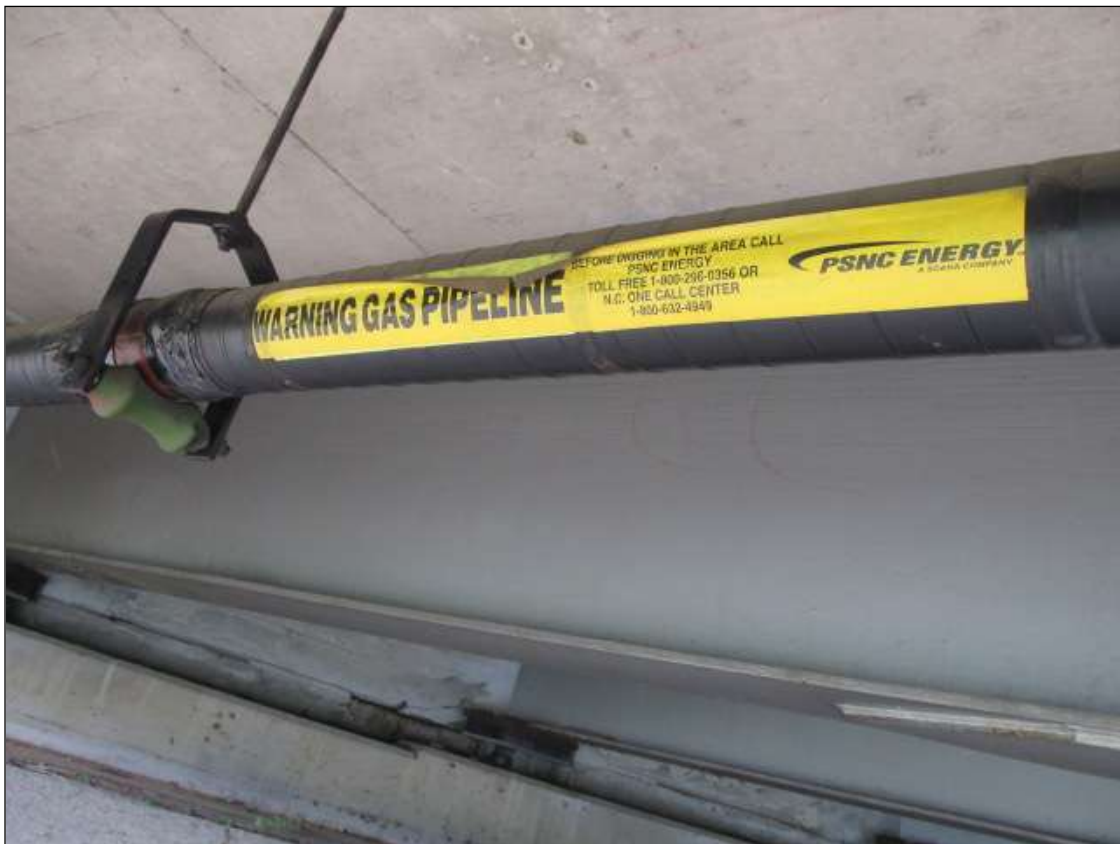
GAS UTILITY UNDER SPAN 5 PHONE INFOR.
