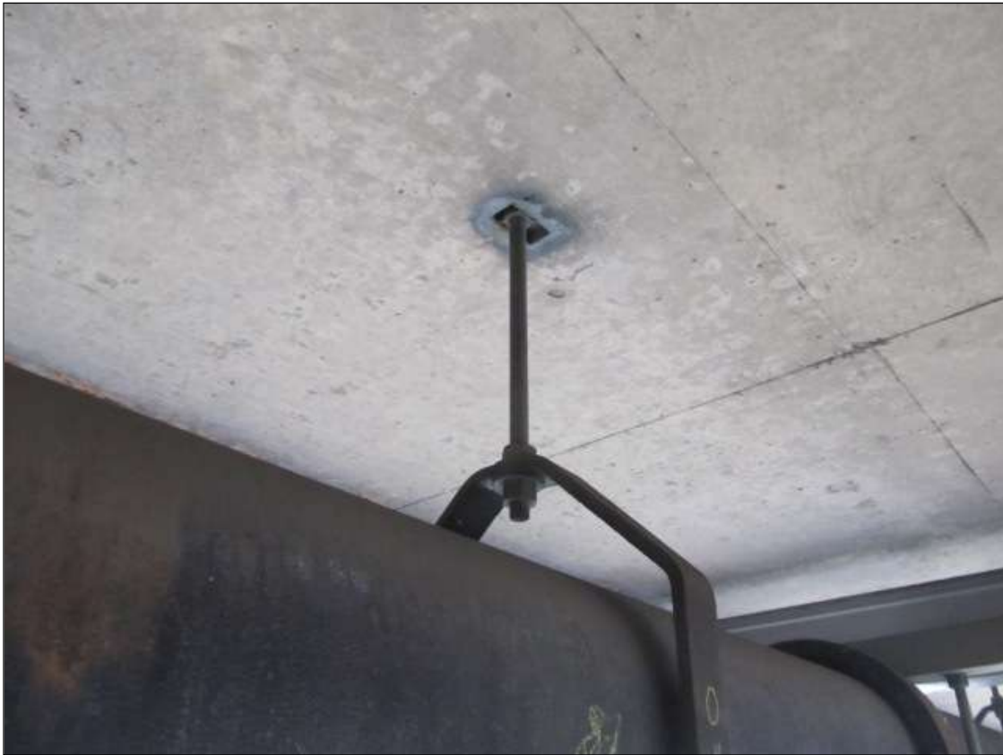
UTILITY HANGER IN BAY 1
