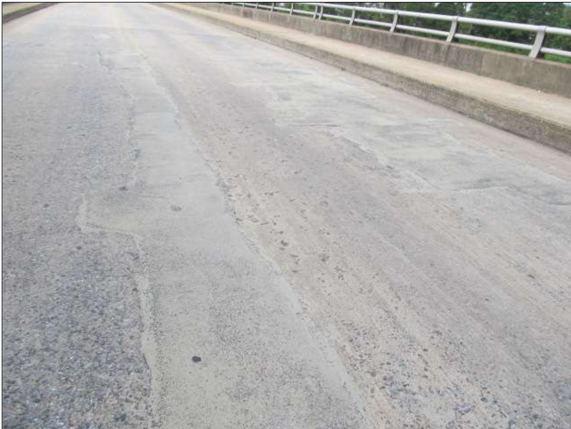
SPAN 1 HAS EPOXY TYPE REPAIRS ALONG THE CL OF RDWY. AND IN THE RT. LANE FOR MOST OF THE SPAN LENGTH.
