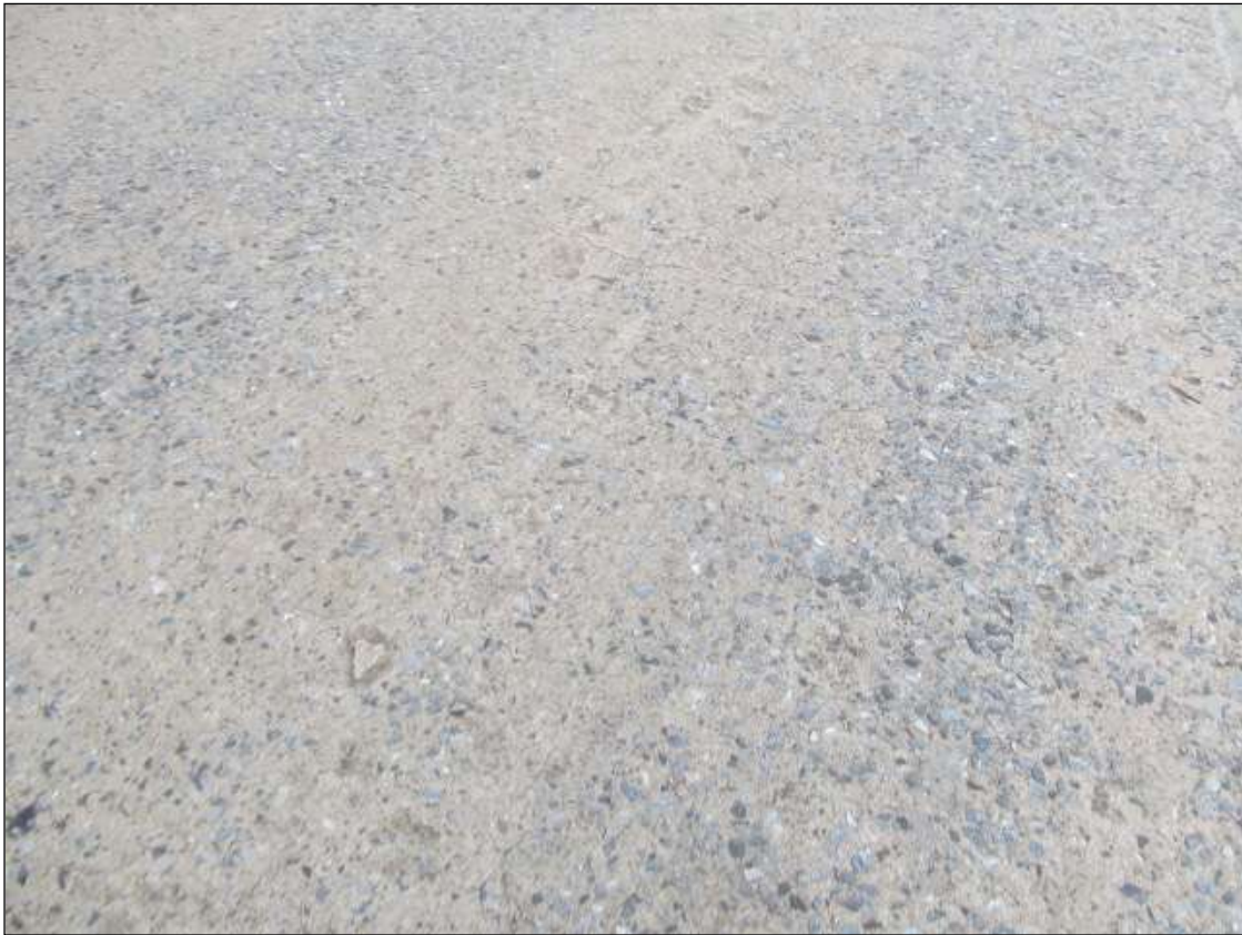
DECK ROADWAY SURFACE HAS SCATTERED DIAGONAL CRACKING ALONG THE JOINTS AND MODERATE MAP CRACKING. ROADWAY SURFACE HAS NUMEROUS POPOUTS AND TRANSVERSE C
